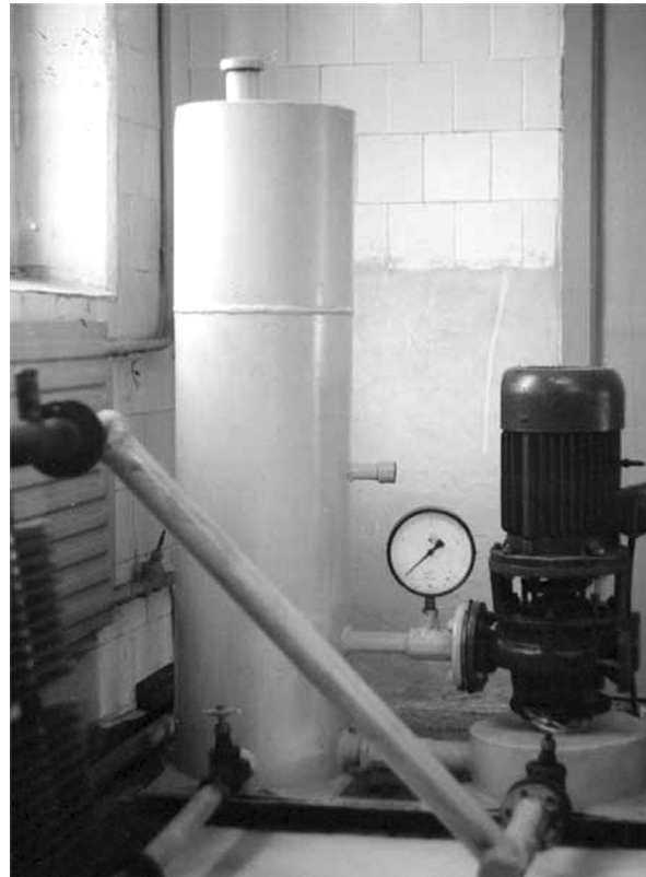
Fig.5 A storage-type TMG thermogenerator
