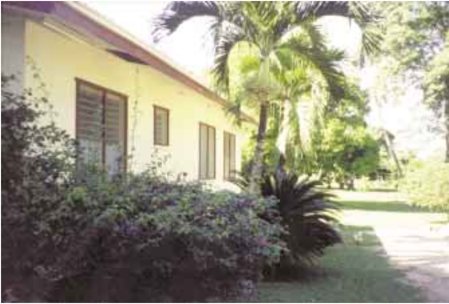
Louvered "jalousie" windows are coated with a reflective surface to block sun. They also readily facilitate ventilation.
