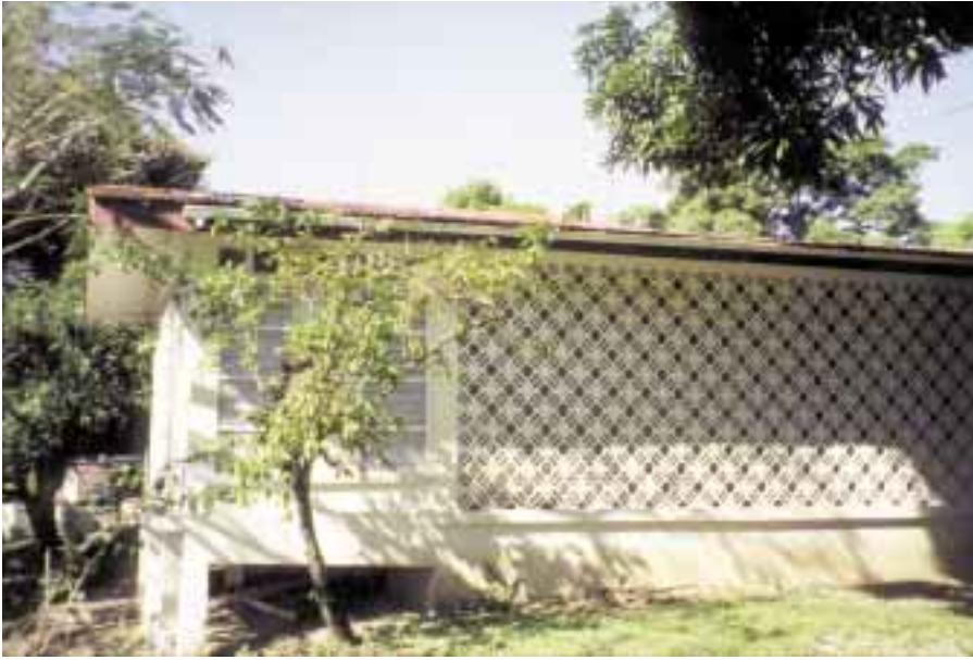
A wall of decorative concrete block allows ventilation and provides shade, transmitting only muted light.
